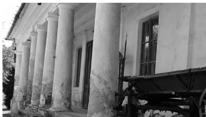
Conacul Ion Pillat, 2019
