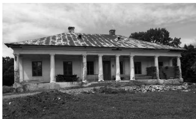
Conacul Ion Pillat, 2014
